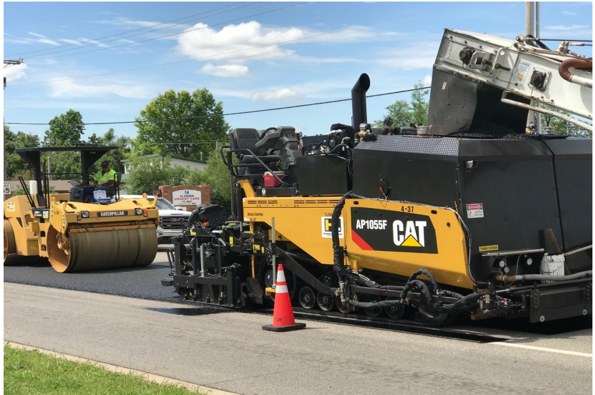
Haskell Lemon Construction Co. lays asphalt on a beautiful spring morning.
